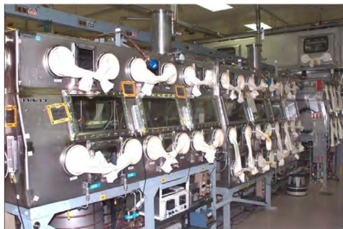
FIGURE 3-23 | AQUEOUS PROCESSING GLOVEBOX LINE AT LANL
