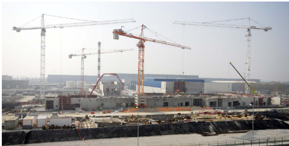
Fig. 17. Georges Besse II plant under construction, March 2007. 54
