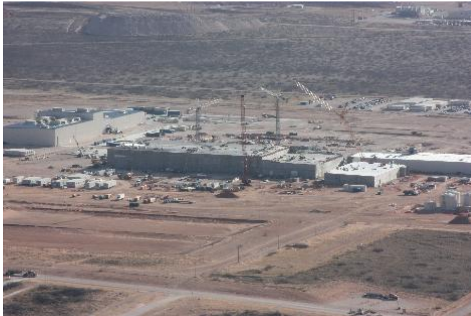
Fig. 7. NEF under construction in March 2009. Source: urencocom
