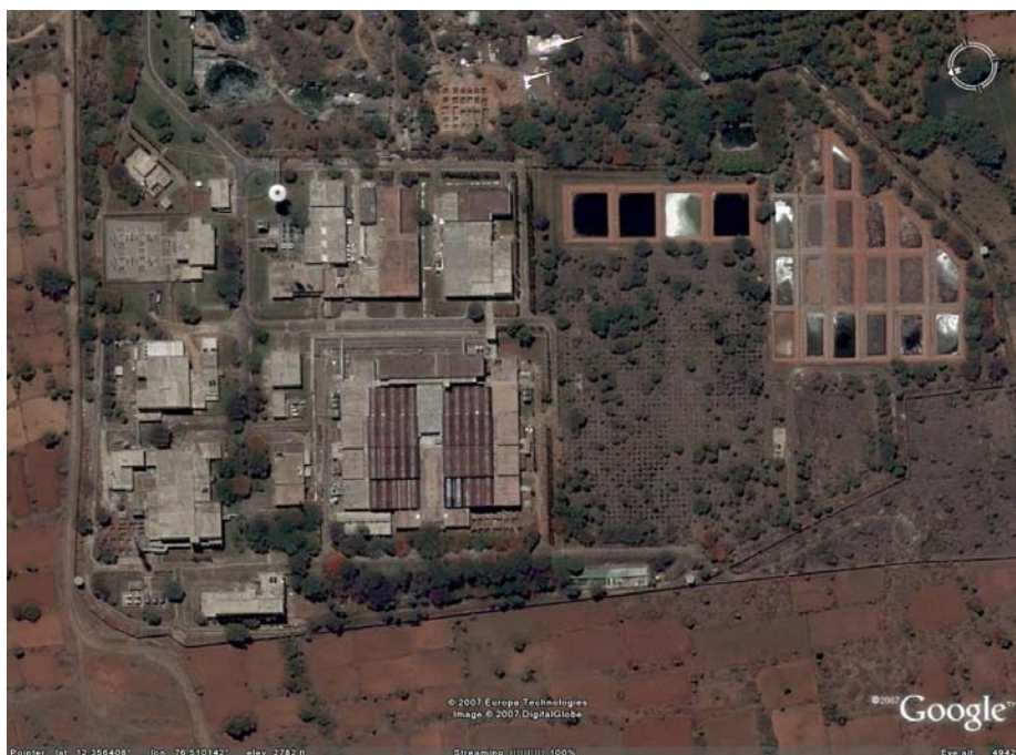
Fig. 37. Rattehalli Rare Materials Plant, India. Source: Google Earth
