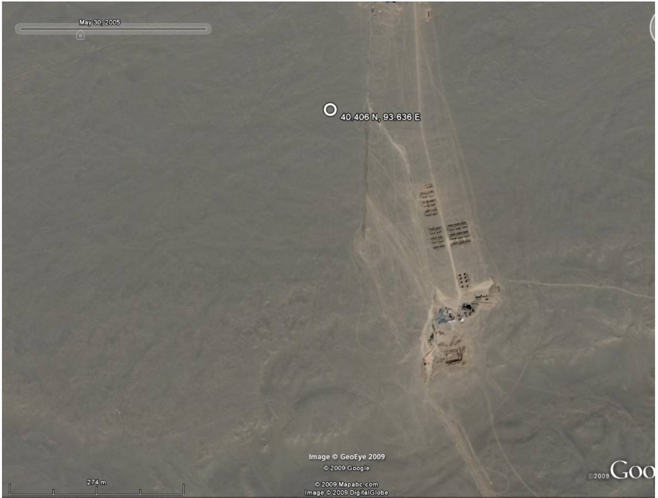
On 2005-05-30 preparations for construction are well along.
