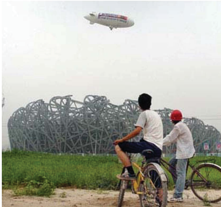
Figure 3. (U) Chengdu Airship ST-3 flying over the Beijing Olympic Stadium's Bird's Nest during construction phase - 10 Aug 2006. 11
