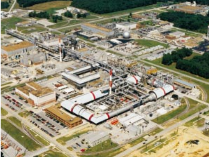
Figure 15-7: The exterior of a large wind tunnel showing the closed-loop circuit for continuous airflow.
