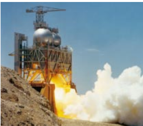
Figure 15-13: A single liquid rocket engine vertical test stand.
