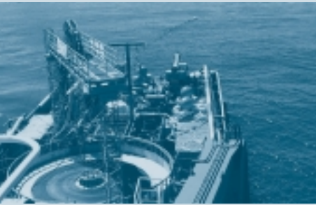
DEPLOYING UNDERSEA CABLE, HYDROACOUSTIC STATION 8, BRITISH INDIAN OCEAN TERRITORY, UNITED KINGDOM
